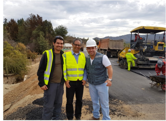
Mauricio, Seirgei and Marco Diaz on the construction site
