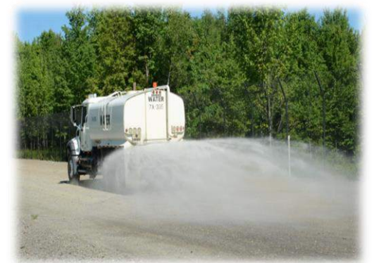
Water spreading
