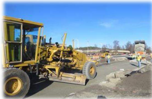
Slope finishing
