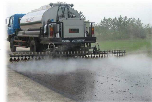
Bitumen emulsion spreading
