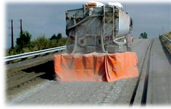
Cement spreading
