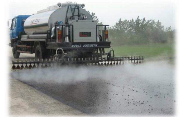
Bitumen emulsion spreading
